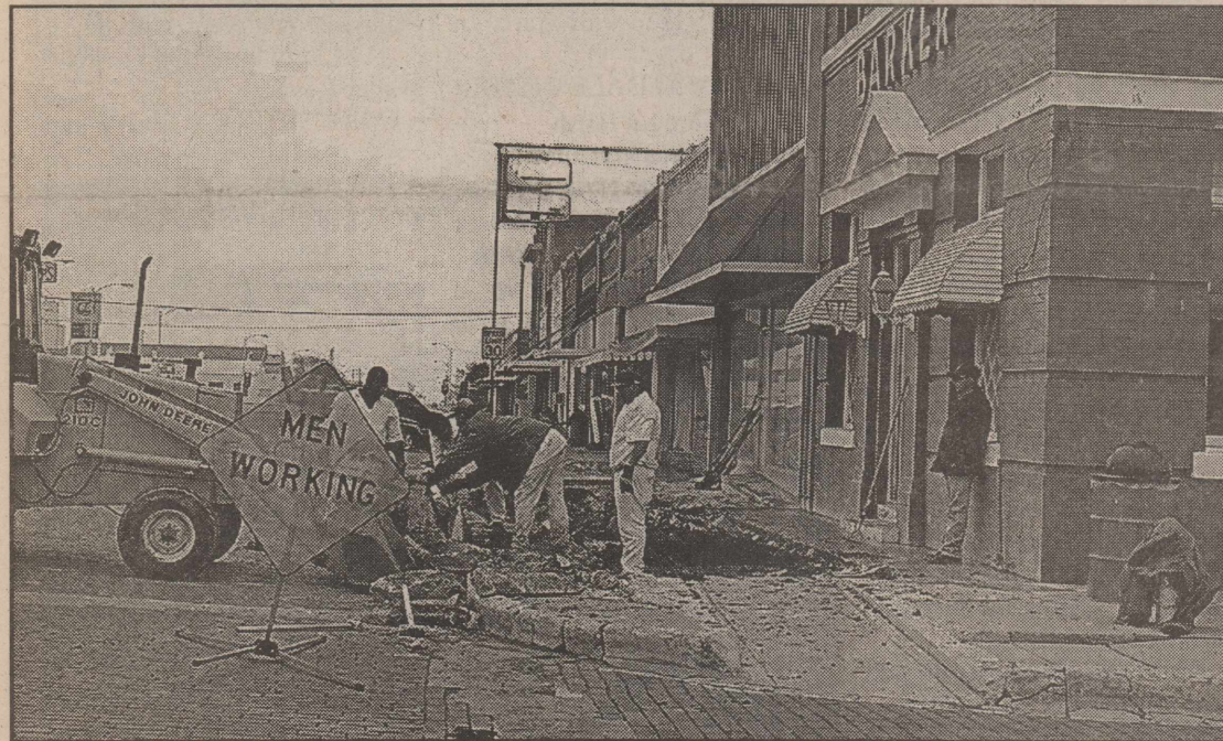
SIDEWALKS IN LOCKNEY ARE NOW BEING TORN UP FOR NEW CONSTRUCTION
