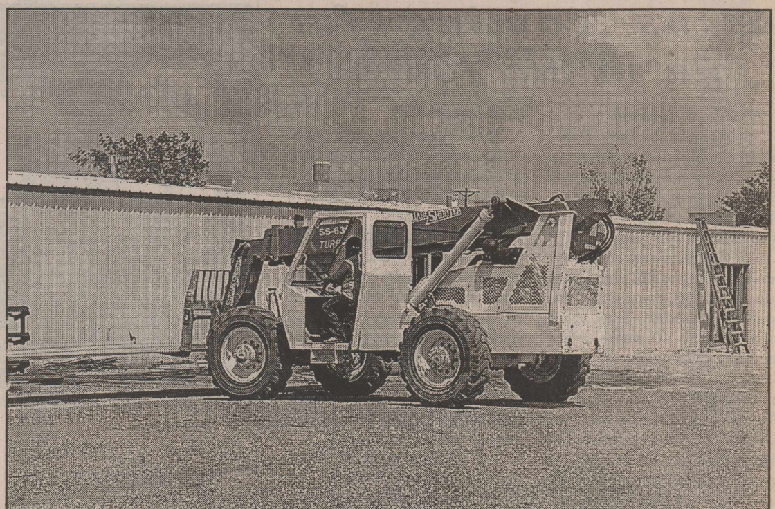
CONSTRUCTION WORK CONTINUES on Lockney's Longhorn Field House. Staff Photo
