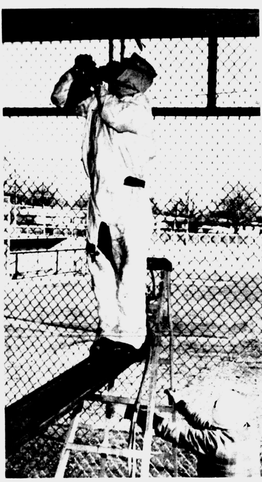
GETTING IT READY — Painters with Arrow Construction Co. took advantage of the warm, sunny weather Friday afternoon to paint the stands at Moffett Field. Major improvements have been made to the field recently to make it one of the best high school facilities in the state. Here, Jose Cabrera sprays the roof of the stands while Serafin Ornelas steadies the ladder for him. (SDN Staff Photo)
