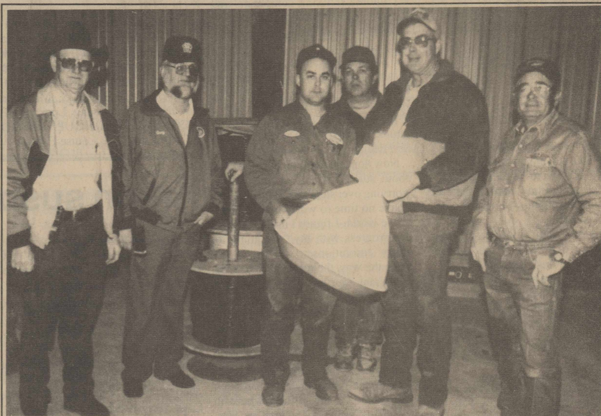
WORKING TOGETHER --Checking out the large lights that are being installed at the Unity Center are: (l-r) Site Foreman Jon LaBaume, Project Coordinator Gary Brown, Brian Polson, of Lubbock Electric, electrician Brent Sanders, Weldon Emert, of Emert Electric, and building contractor Ed Marks.
