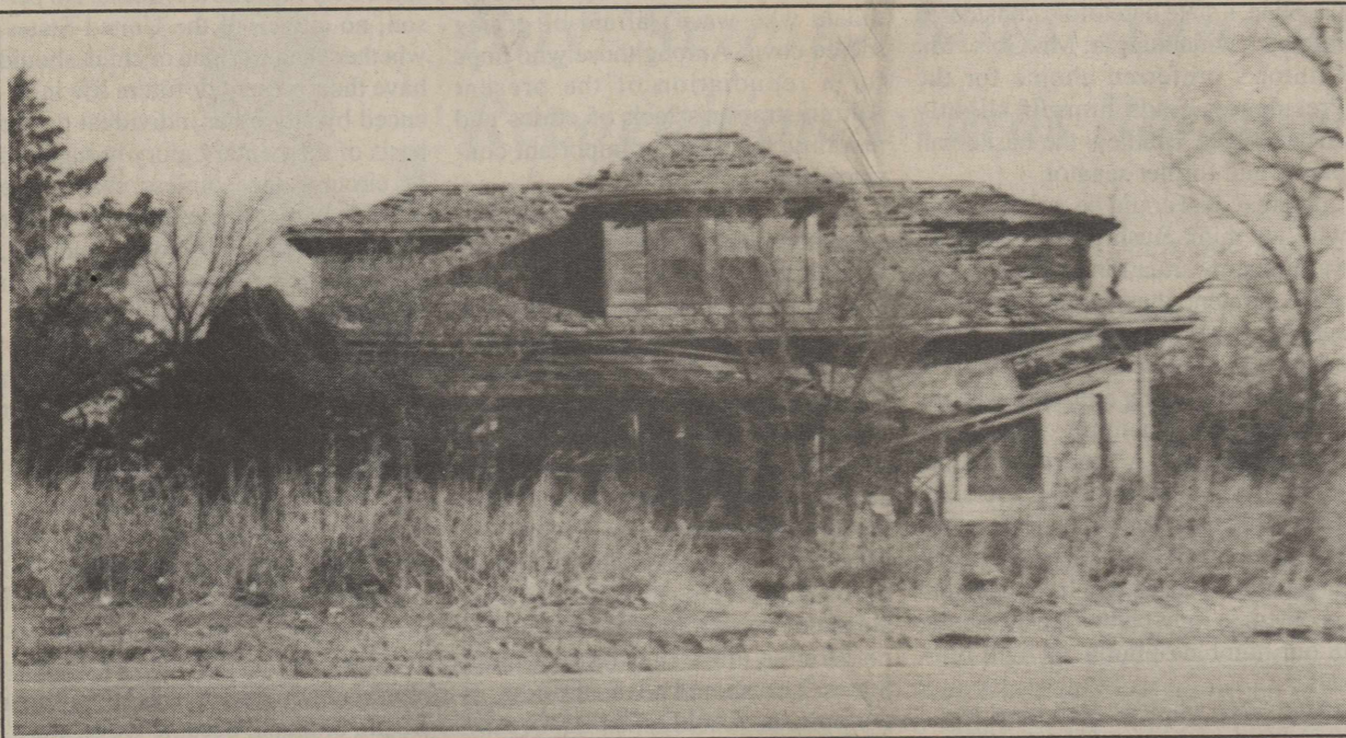
LOCKNEY LANDMARK TORN DOWN
