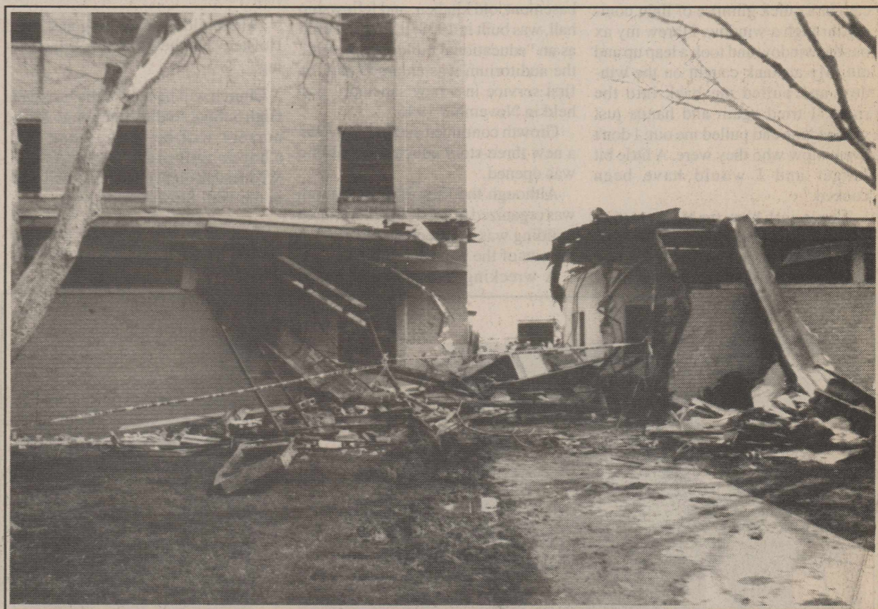
THE BREEZEWAY BULLDOZED TO SAVE MAIN AUDITORIUM-Firefighters Sunday night, March 12th, ran a bulldozer between the buildings of the First Baptist Church in order to save the main Sanctuary. The devastating fire destroyed the old auditorium and the Sunday School building. Staff Photo
