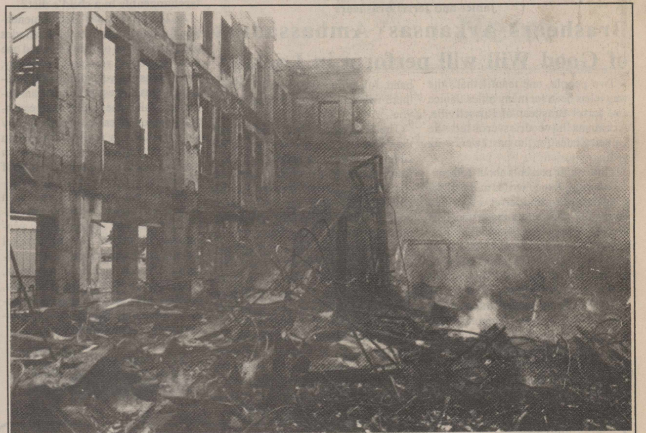
THE SMOLDERING RUBBLE -The ruins of the First Baptist Church Sunday School building were still smoldering Monday morning after the devastating fire Sunday night. Three floors fell into the basement area as shown in photo. (see related story) Staff Photo
