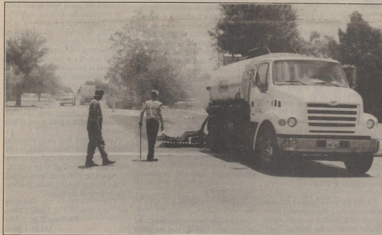
TOPPING THE STREETS-Crews were out in full force last Thursday seal-coating many of the Floydada city streets. Gravel was added on top of the hot tar to finish the project. Staff Photo
