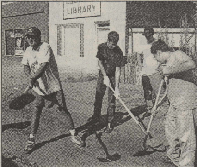
EAGLE SCOUT PROJECT--Will O'Connell (center) is helped with his Eagle Project by fellow Scouts. O'Connell is working to replace the sidewalk next to the old Library building.
