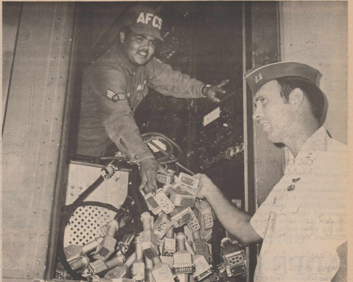
CABLES, CABLES — Sgt. Pedro Paradez and Capt. Kelly Cartron, 1958th Communications Squadron, unit at Terry County Airport. (Courtesy photo) straighten some of many cables that were unplugged
