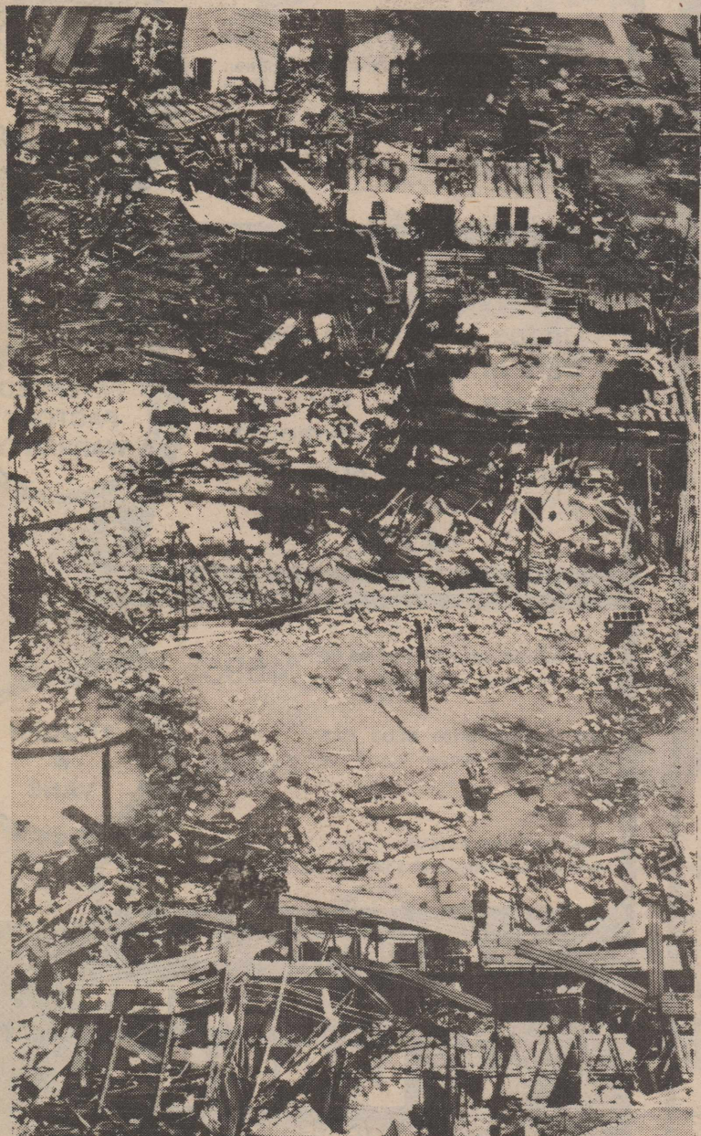
Destruction in Lubbock after '72 tornado.
