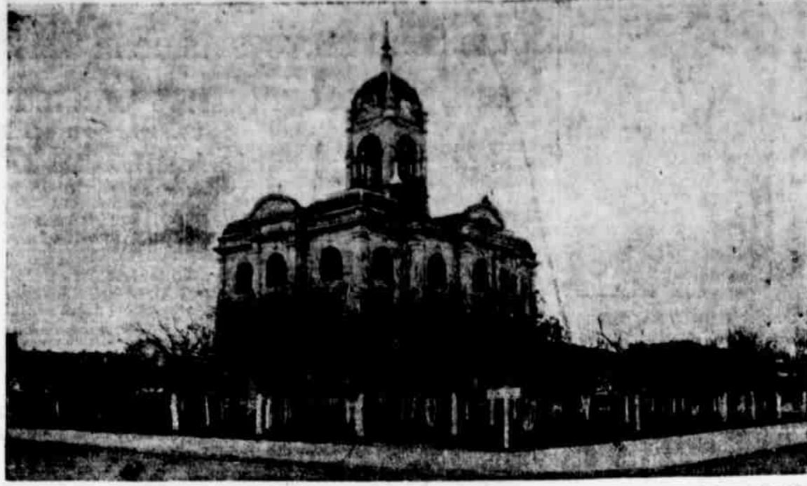
Haskell County's first permanent courthouse building, shown here, was erected in 1890. It was one of the most pretentious structures of its kind in this section and one of the largest. From the tower which surmounted the three-story building, the country could be viewed for miles. A
