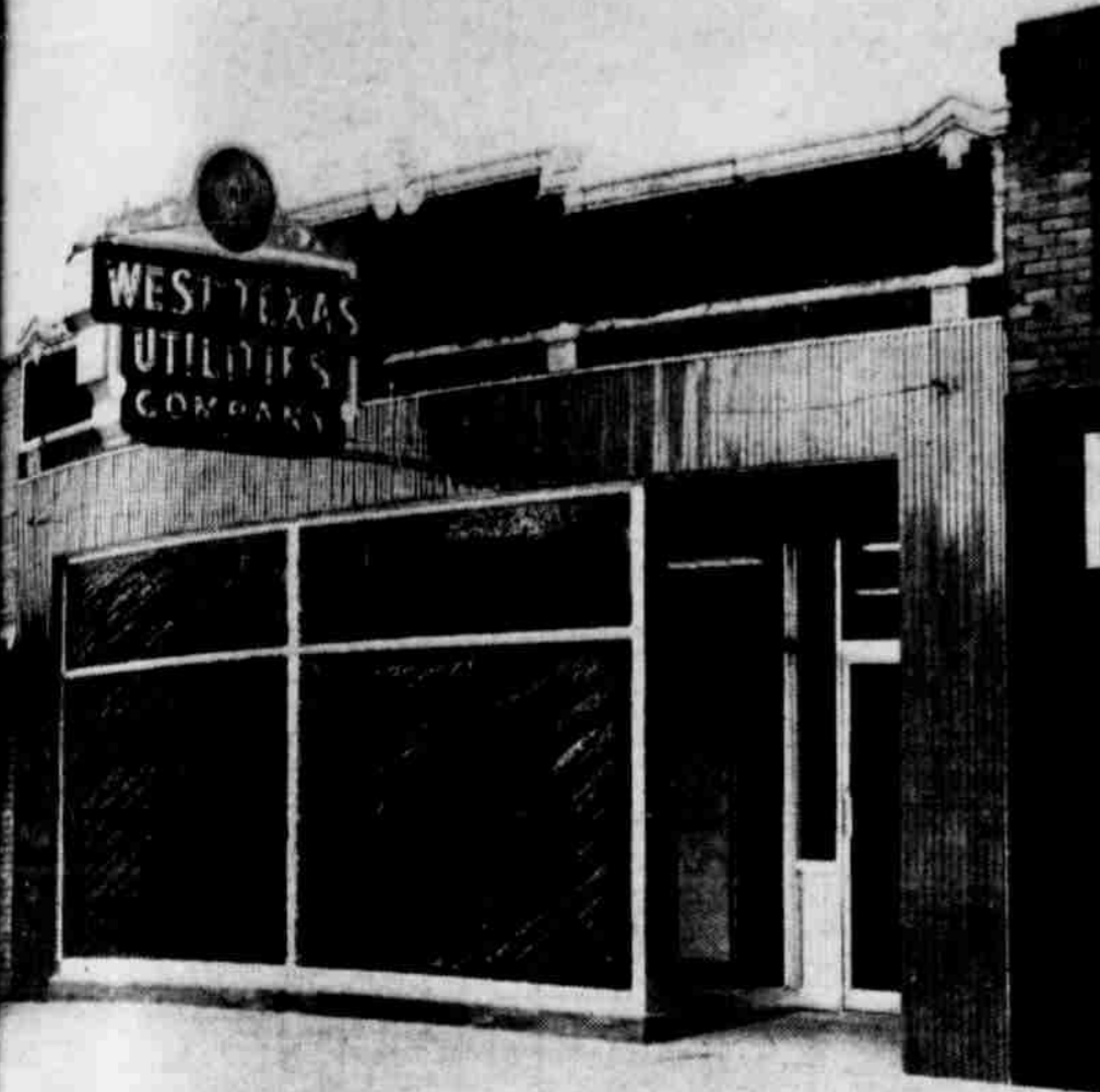
Haskell Local Office just recently remodeled with an entire new front which is in keeping with the appearance of the south side of the square.
