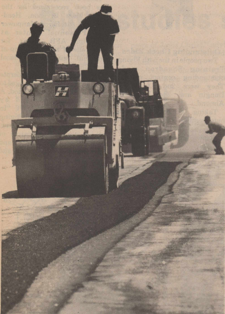
SrA Terry Cox and A1C Nick Marquez (sitting) roll the new asphalt into place while other CE workers follow with a giant vacuum cleaner. In the background, TSgt. Steven Cofield makes sure the cleaner doesn't run onto the fresh asphalt. At right, Amn. Wayne Wright spreads some of the smoldering asphalt in place.
