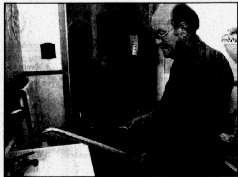
Bob Elwood, with Ellwood Enterprises, shows Maria Mendoza, 110, the safety rail that he is installing in her bathroom. Community and Senior Services is having the safety equipment installed for Mrs. Mendoza.
