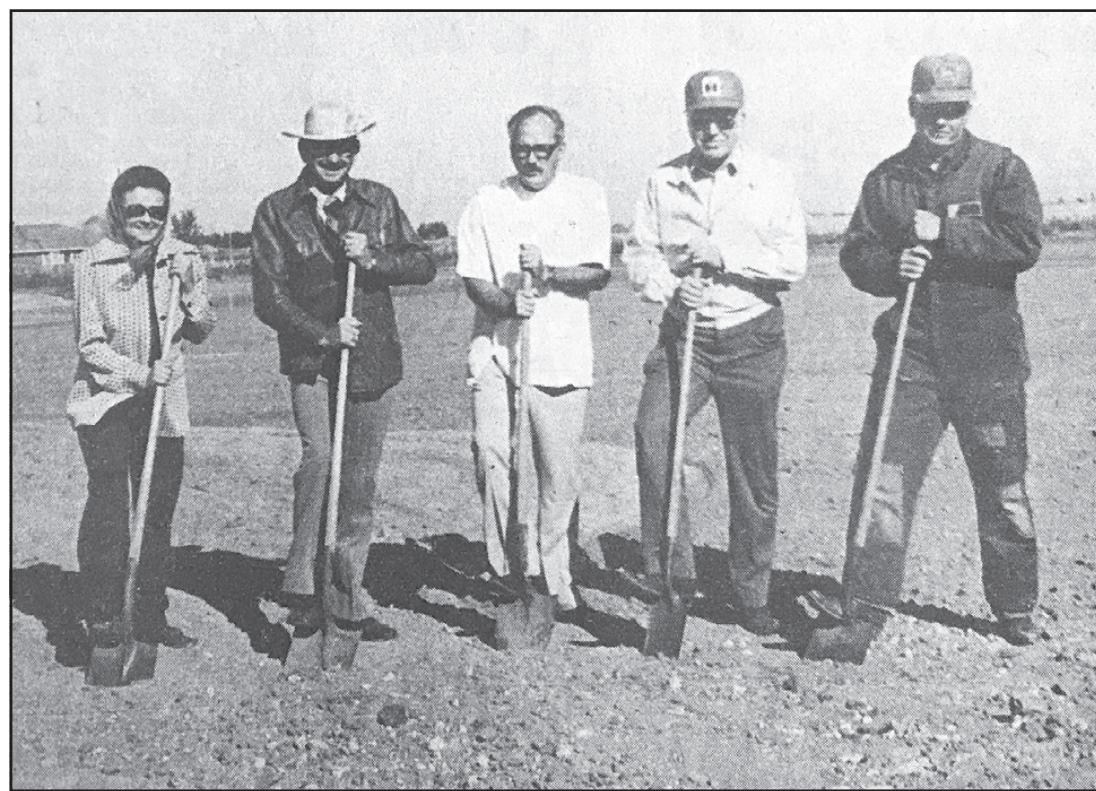
BREAKING GROUND.... An official groundbreaking ceremony was held at the Friona Nursing Home site Tuesday morning. Left to right are June Spring, mayor R.L. Fleming, Dr. Bob Alexander, Andy Hurst and Delton Lewellen, contractor. Lewellen has estimated the job to take nine months to complete, and says he might beat that estimate if the weather is favorable. (Friona Star, Sunday, November 2, 1975)
