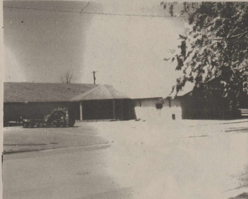
The Assembly of God Church in Stratford is getting a new look. If you haven't seen it drive by and take a look at their new addition. The church members are very proud and it looks very nice from the outside.
