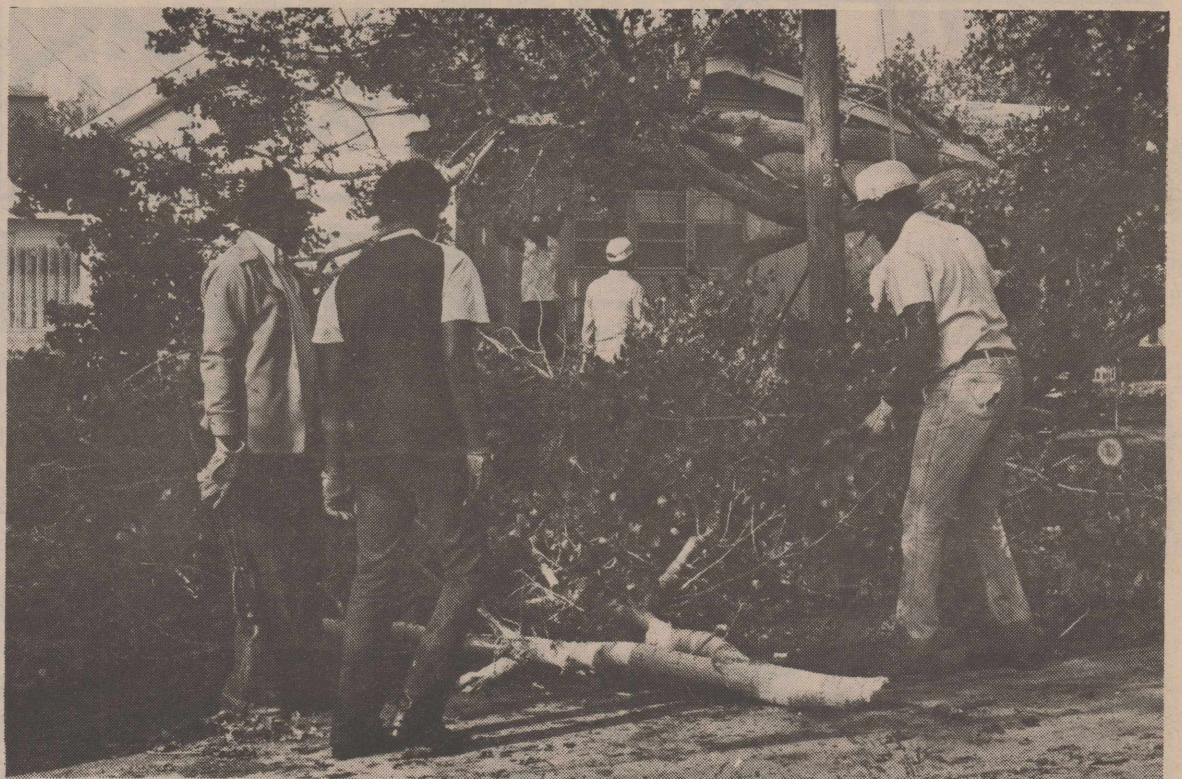
Clean up begins in housing
