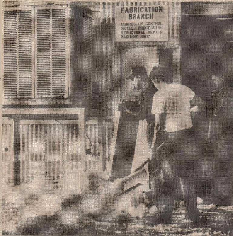
Another damaged air conditioner
