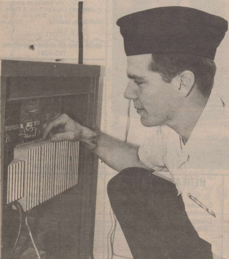
SSgt. Mark McSorley inspects the Intrabase radio Transceiver.
