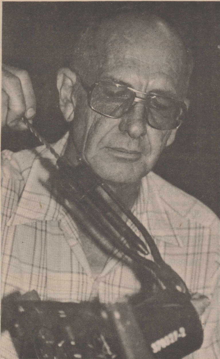
Charles Butler safety wires an MA1A tachometer.
