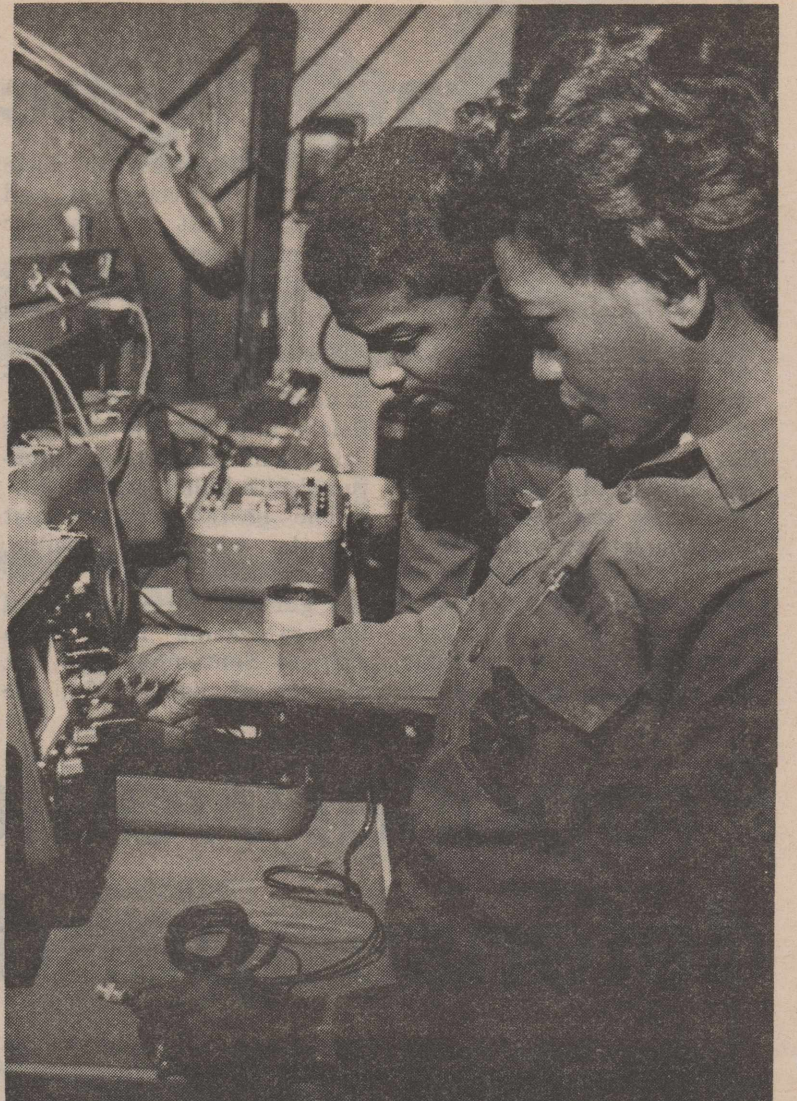
Non-Destructive Inspection Specialist SrA. Sammie Sykes and NDI Technician SSGT. Arturo Beltran calibrate an ultrasonic unit to detect subsurface defects in the T-37 carrythru spar. Both are assigned to the 64th Field Maintenance Squadron's Non-Destructive Inspection shop.
