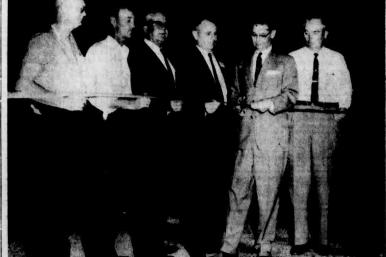
Cal Young president of West Texas Utilities Company, snips a ribbon officially opening to traffic the new stretch of paved road to WTU's Paint Creek Power Plant.
