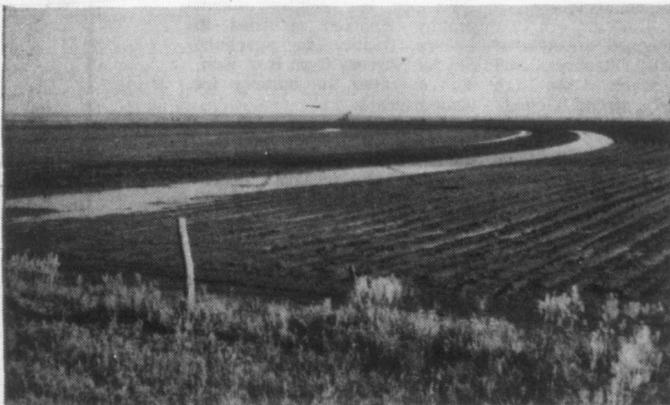
The construction of terraces and diversions is an excellent way to control and stop erosion on rolling land and sloping cropland. With terraces and diversions, rainwater is channeled across the field to a suitable outlet such as a grass waterway or pond. Through this channeling action, water is transported across the field and isn't allowed to cut down across the field, stopping erosion and the development of gullies.
