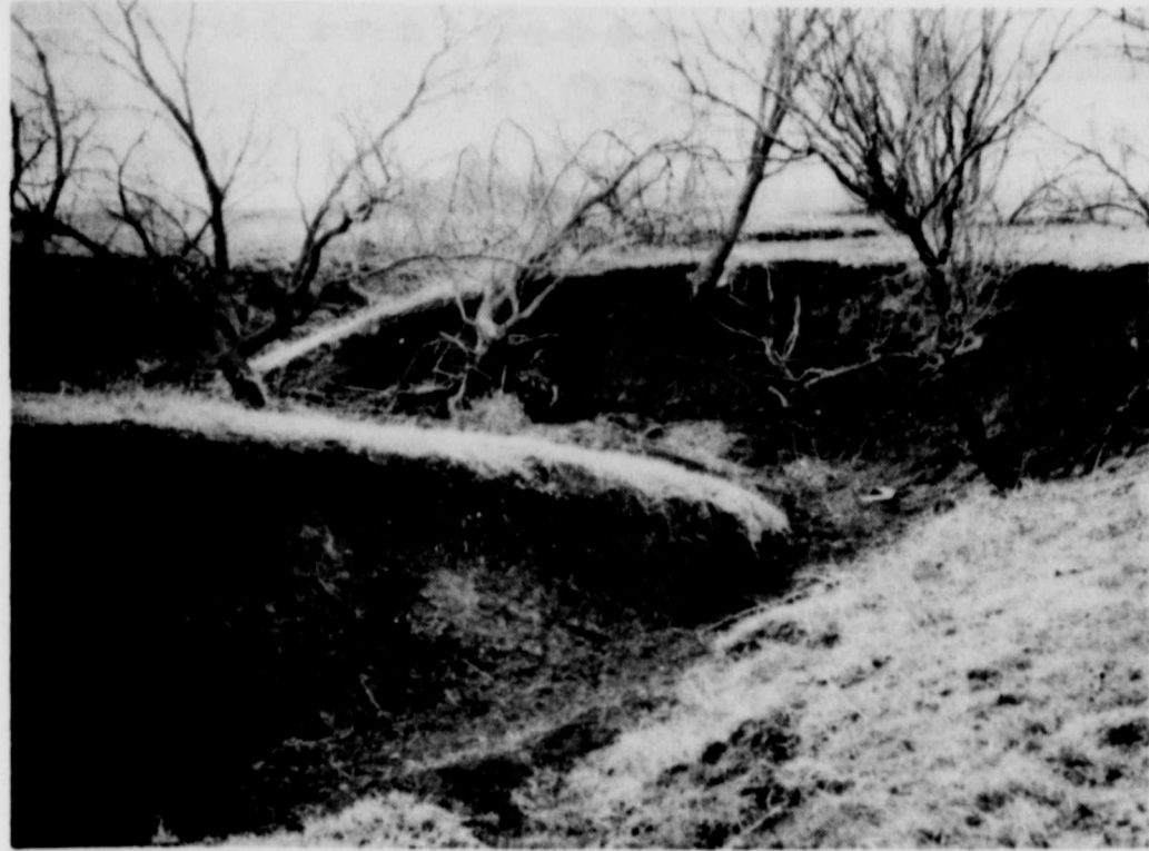
ELECTRA, TEXAS---EROSION---An active gully in need of critical area shaping and planting on the Dewey Dovel farm, 10 miles southwest of Electra. (USDA--Soil Conservation Service Photo by William H. Lewis, Jr.)
