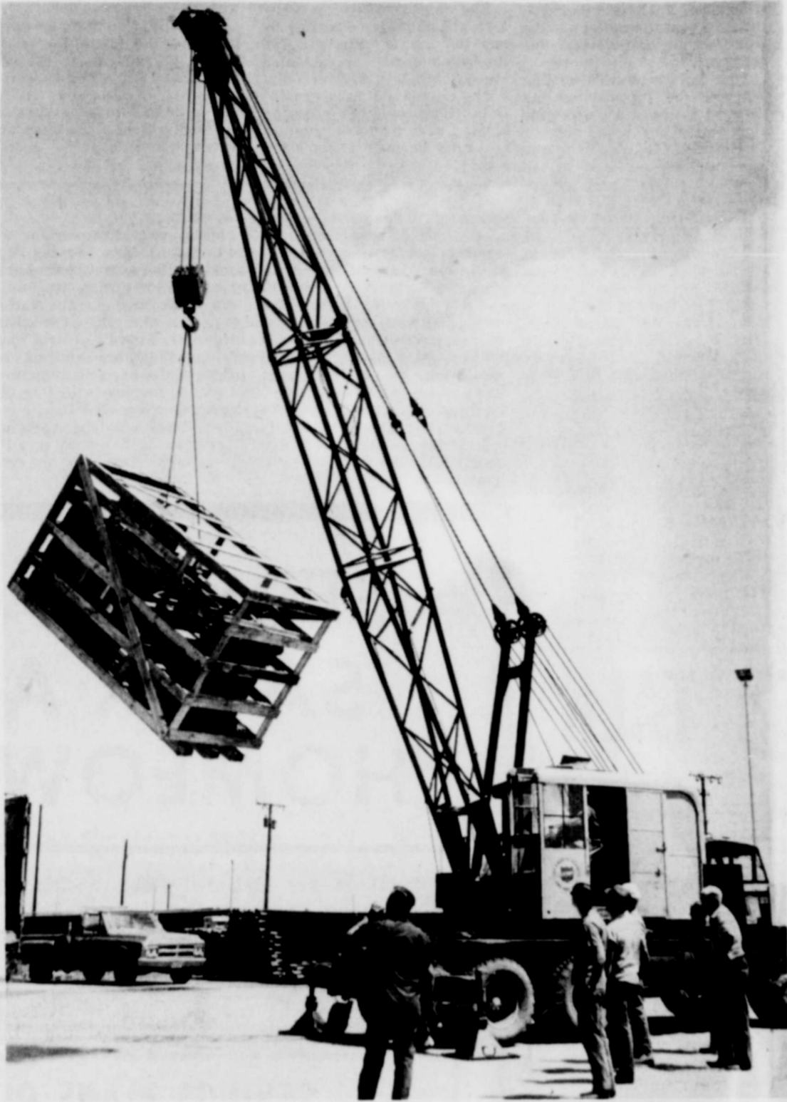
UNLOADS HYDRAULIC PRESSES--Huge crane is shown as it unloads one of two 35,000 pound hydraulic presses received by CIBA Pipe Systems, Friday.
