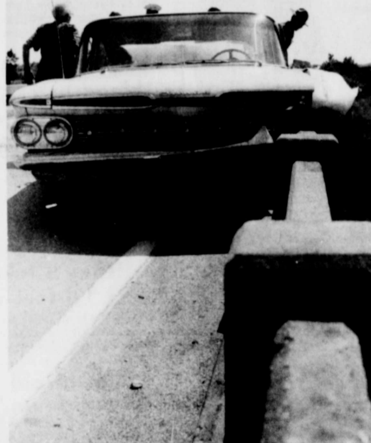
CAR RIDES RAIL--The 1959 Chevrolet, above, rode the rail of the Red River Bridge for 1,000 feet before coming to a halt in a Tuesday evening accident.
