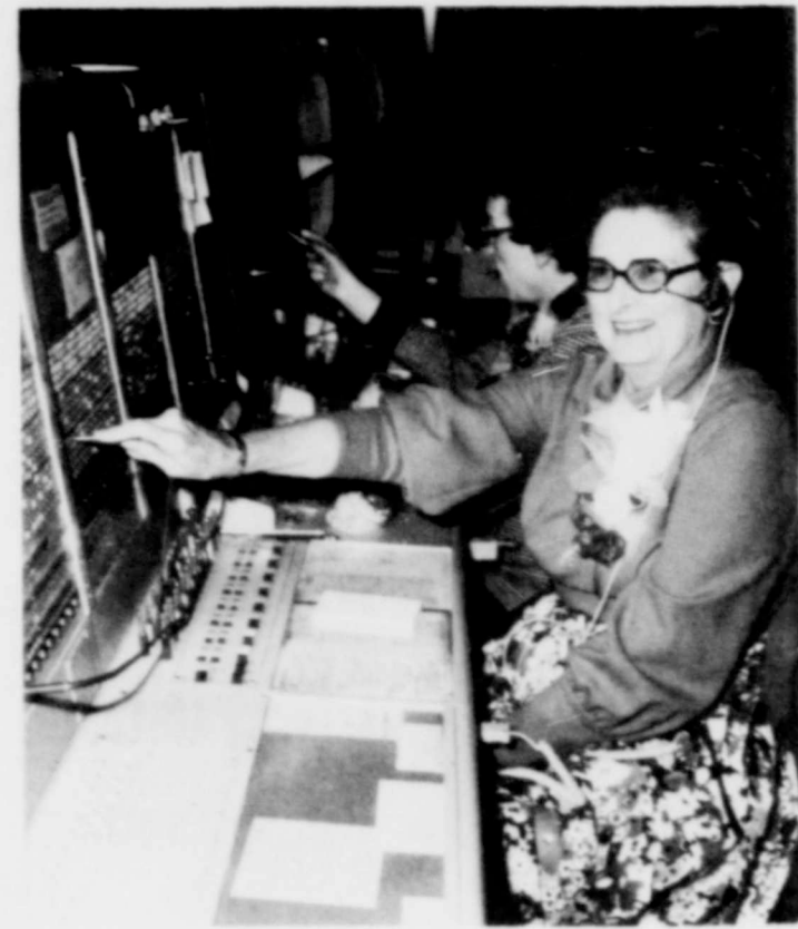
SHEPPARD AFB, TEXAS--SHEPPARD'S CHIEF OPERATOR RETIRES--Mosselle Gay, chief operator at Sheppard Air Force Base for more than 23 years, makes one of her last switchboard connections at Sheppard Air Force Base as chief telephone operator. She retired Friday and will live in Burk Burnett, Tex. (OFFICIAL USAF PHOTO BY TS/SGT. ROBERT PAGE)
