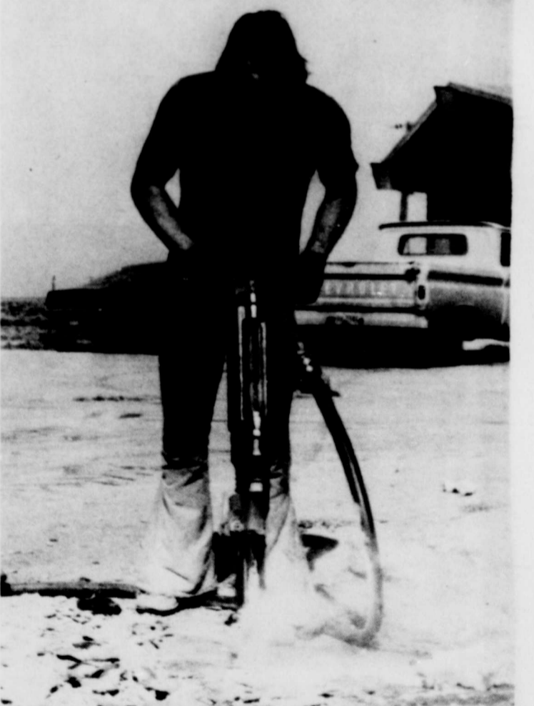
Even Jack-Hammers work for new Burk water line.
