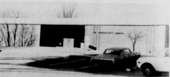
LIBRARY BUILDING--An outside view of Burk Burnett's "House of Knowledge" is pictured. The location is 215 East Fourth in downtown Burk Burnett. The Burk Burnett Library has over 13,000 volumes. (Informer/Star Photo)
