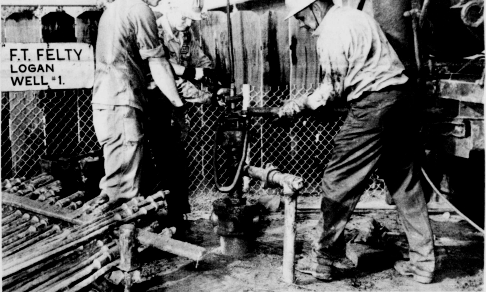
ERA IN LOCAL HISTORY COMES TO END —An unforgettable era in Burk Burnett's history came to a close Monday as workers pulled the rods and tubing from the last oil well in the city limits of the old original oil boom days. F.T. Felty Well #1 pumped its last barrel of oil last week as workers began pulling the well Monday morning. The well was drilled in 1918 and produced
