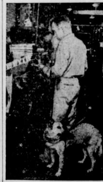
Charles A. Kime, a jig-builder in a Burbank, Calif., aviation plant, lost his sight in an accident. Now he is back at work in the same factory, and is pictured here installing rivet nuts for the de-icing boot on the leading edge of P-38 empen-
