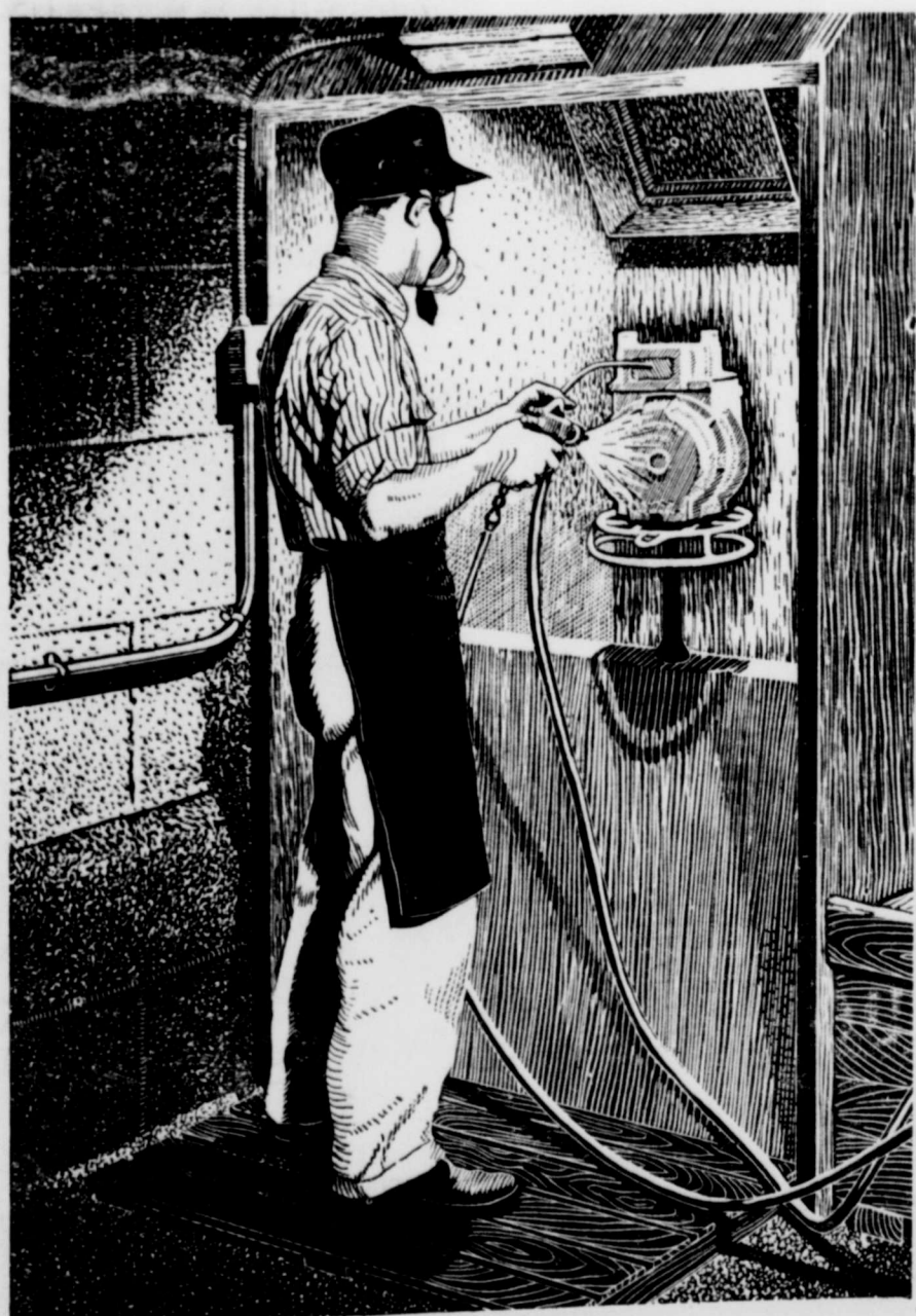
Equipment maintenance is an important factor in dependable natural gas service.
