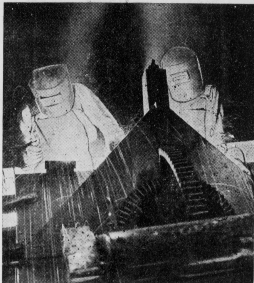
This picture is typical of the way the national defense program is progressing. Here two hooded welders at the plant of the American Car and Foundry company in Berwick, Pa., are shown at work on some of the armor plate that goes on the fighting tanks being turned out by the hundred. Tanks roll off the assembly line at a rapid rate.
