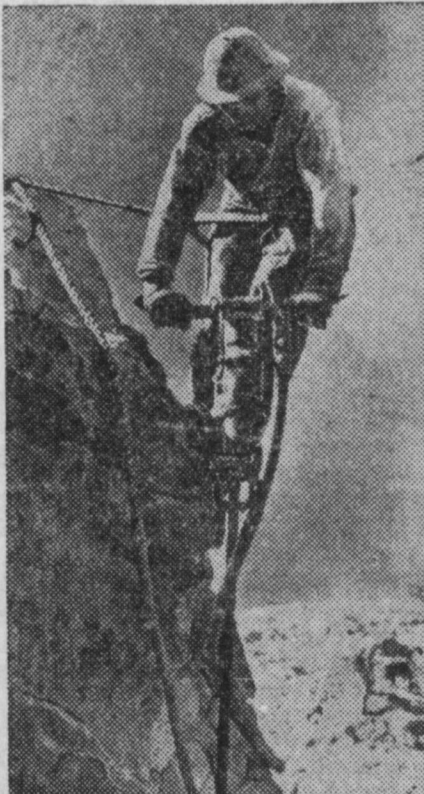
Men who work to increase our supply of electric energy are soldiers, too. Photo shows a jackhammer operator drilling a hole for a dynamite blast on an abutment of Shasta dam, near San Francisco, Calif.
