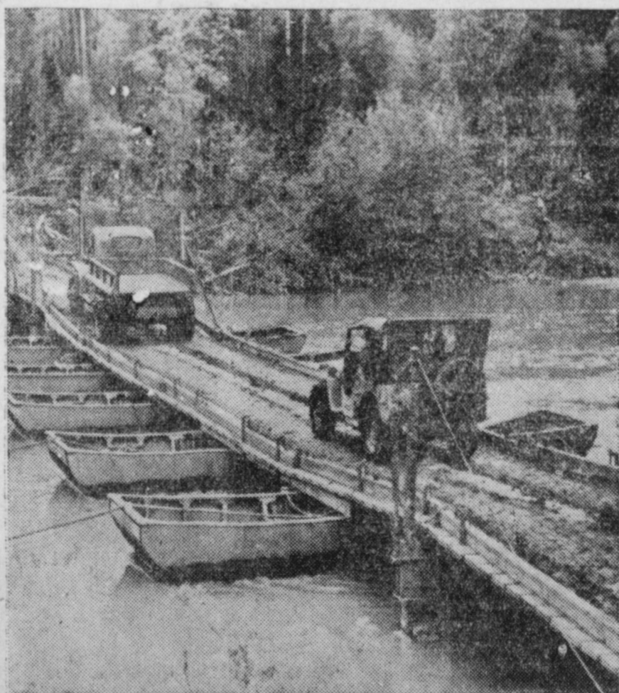
The Alaska highway, which is being rushed to completion through virgin forests on the east side of the Rockies, will make a military road protected by a chain of coastal mountains from the Pacific Northwest to our Alaskan defense area. Photo shows a pontoon bridge over a river. Substantial loads of equipment and supplies may be moved freely over this type of bridge.
