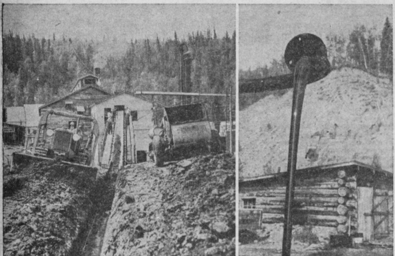
Ten thousand square miles of prehistoric, mineral-rich oil sands in Alberta, Canada, will provide the United Nations with huge quantities of oil. Experimental production has been in effect for more than a year at McMurray, 300 miles northeast of Edmonton. Photos show (left) conveyor belts carrying oil sands to the separation plant where, through flotation, hot water washes oil free from sand. Right: "Black gold" flows freely through the pipeline after the separation process is completed.
