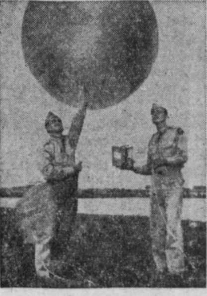
The two men are about to release a radio-meteorograph. This little instrument when carried aloft by the balloon will transmit radio readings of pressure, temperature, and humidity to a station below. There is also a parachute attached to bring the instrument back.
