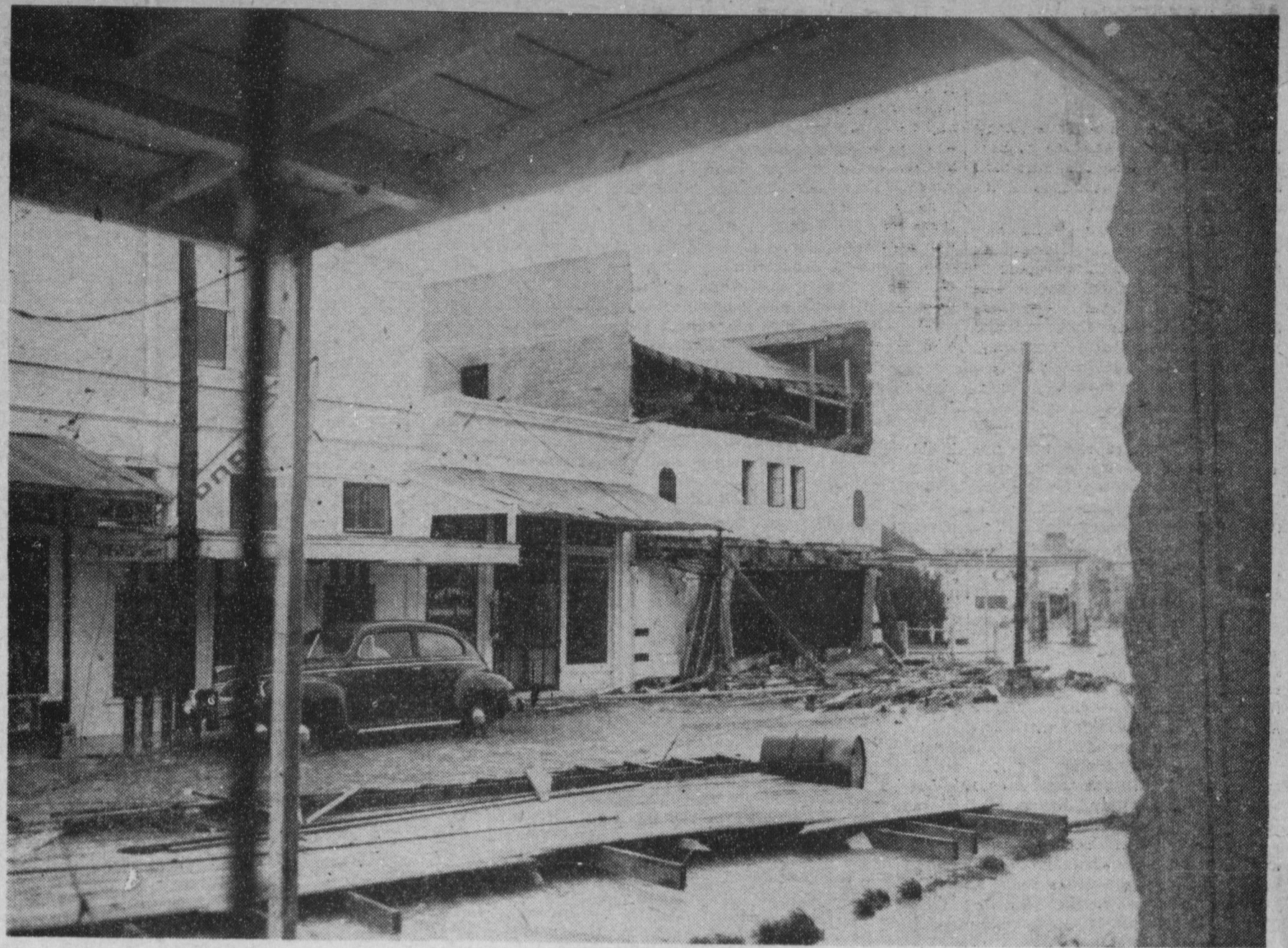
MORE SERIOUS DAMAGE: —Port Lavaca took one of the hardest blows in the storm. This street scene shows how most of the down town area of the town looked like late Monday afternoon. Most of the shrimp fleet is out of commission and the job of reconstruction in all parts of the town will be huge.
