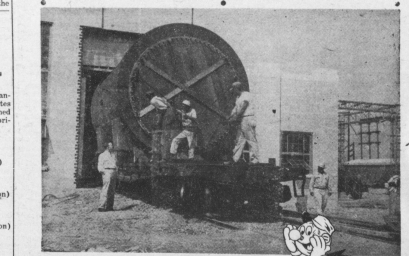
A huge, new condenser for La Palma Power Station's Number 5 generating unit is shown upon arrival at the San Benito plant. This is only one part of the 20,000 kilowatt generating unit, which is expected to be in operation early next year.
