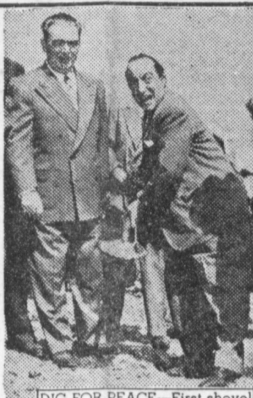
DIG FOR PEACE —First shovel of ground broken for new United Nations headquarters in New York City is held by Benjamin Cohen, acting secretary of UN, with Mayor William O'Dwyer looking on. Headquarters buildings will cost $65,000,000.00.
