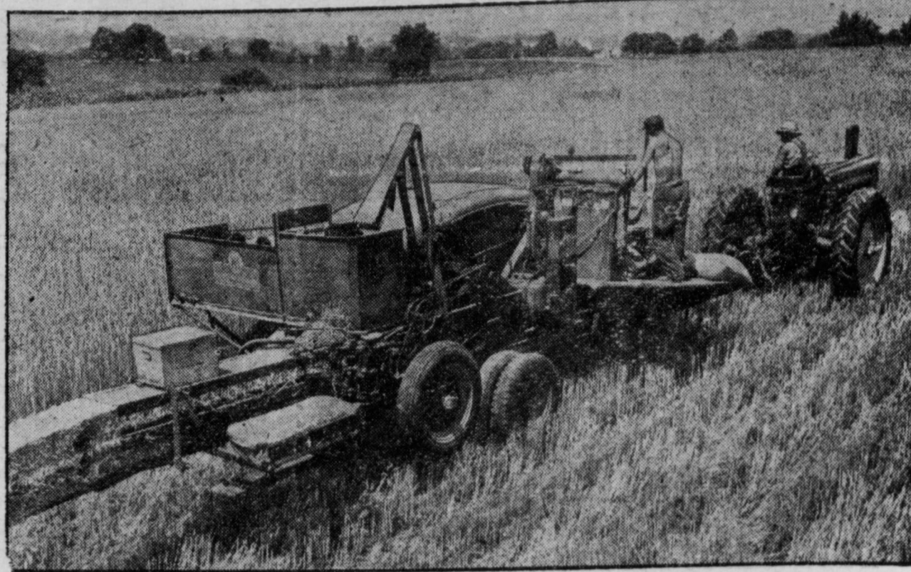
COMBINE COMBINES OPERATIONS —This machine is the latest idea in speeding up the harvesting of the nation's biggest peacetime wheat crops. A standard automatic twine-tying baler was joined with a combine to do several jobs at once. With the arrangement, a two-man crew can cut the ripe wheat, thresh it, bag it, and bale the leftover wheat straw in one continuous operation. At the left an automatically twine-tied bale is shown ready to drop from the baling chamber.
