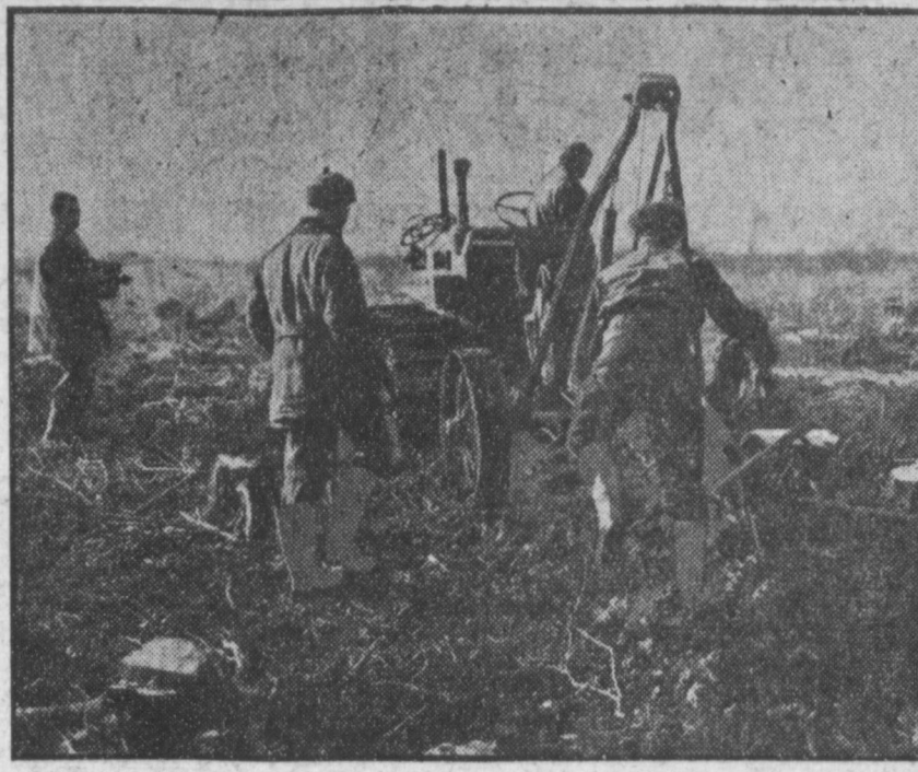
FRENCH RECLAIM SWAMP LAND —Workmen start the first day of work in the reclamation of France's largest swamp, the Marais Vernier, which is 5000 acres. With the help of Marshall Plan aid, the French hope to restore the valuable farmland to use. The swamp is located in the Seine Estuary region in Normandy.
