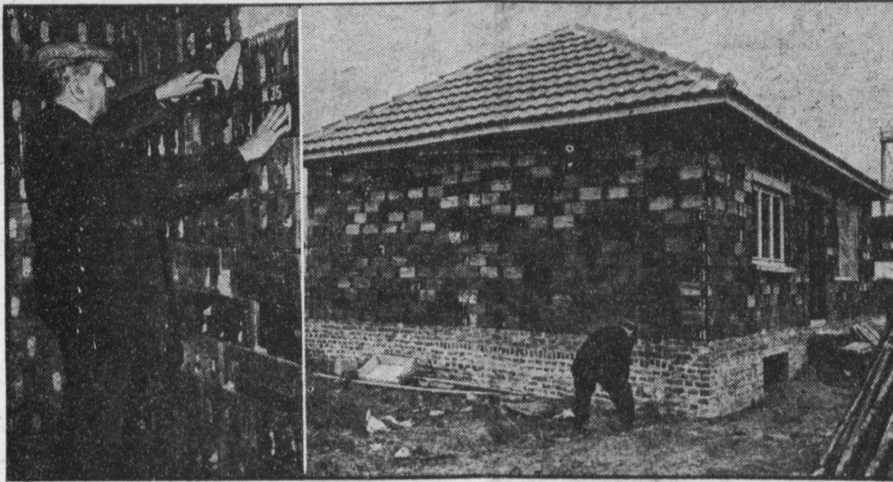
HOME FROM THE WAR —A German architect, turned homebuilder, is shown, left, putting the finishing touches to one wall of the cottage he is constructing in Frankfurt, Germany. Needing a place to live and lacking funds for conventional materials, the builder used wooden ammunition boxes that had been stacked in a former German army depot. To give the boxes the necessary strength to support the roof the compartments designed to hold shells were filled with cement. At right is a view of the outside of the building as the architect caulked basement bricks.
