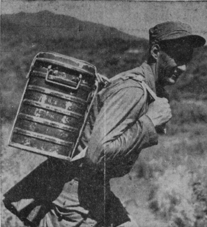
EASING THE LOAD—The soldier striding along with the full food container on his back moves with comparative freedom and ease, thanks to a simplified load-carrying device developed by Army Quartermaster Corps. Light in weight and simple to adjust, the carrier is a seven-foot length of webbing equipped with metal load-spacers and a snap by which it is fastened around the shoulder. It may be used by an individual or a team of two to carry ammunition, machine guns and tripods, mortars and mortar base-plates, rations, water and fuel cans or litter in combat areas.
