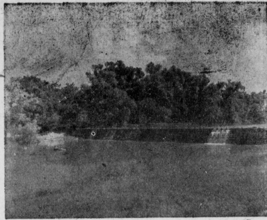
BLANCO STATE PARK on Blanco River at U. S. Highway 281 has a series of picturesque rock dams on the swift flowing stream that was named for the clearness of its water. The park extends along both sides of the river with many good sites for picnicking. A stone recreation building, rest rooms and playgrounds make it an attractive day-use park. Photo Courtesy Texas Highway Department.
