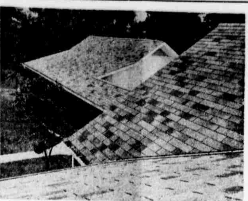
A quality roof, like these heavyweight asphalt shingles, is a good investment because it gives long-lasting, trouble-free service. When choosing a roofing material, look for durability, low-maintenance, appearance, and wind and fire-resistance.
