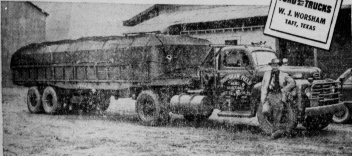
Ford Model F-8 BIG JOB shown here has Gross Combination Weight rating of 39,000 lbs., as a tractor; Gross Vehicle Weight rating of 21,500 lbs.
