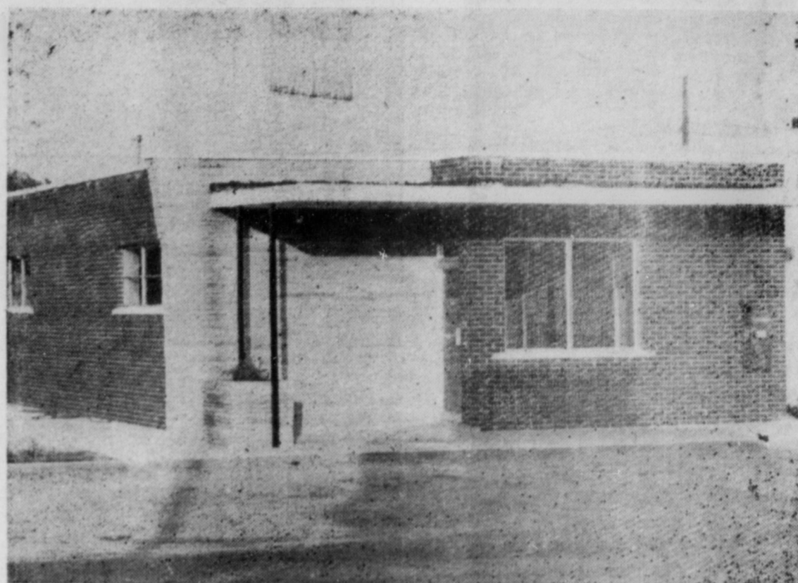
NEW JAYTON POST OFFICE
