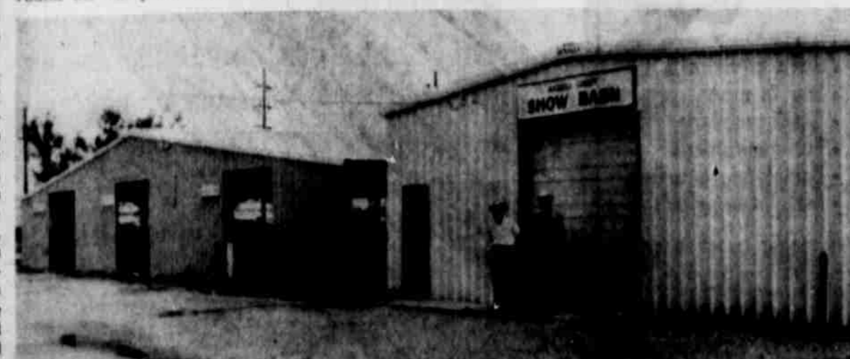
NEW LIVESTOCK EXHIBIT BARN: The Haskell County Fair Grounds have taken on a new look. Pictured with the new facilities is Rex Felker, (at left), Chamber of Commerce Manager, and Executive Secretary-Treasurer of the Haskell County Fair Association, and at right, C. A. Thomas Jr., president. The Fair will get underway Thursday, October 1, for three big days and nights of activities.
