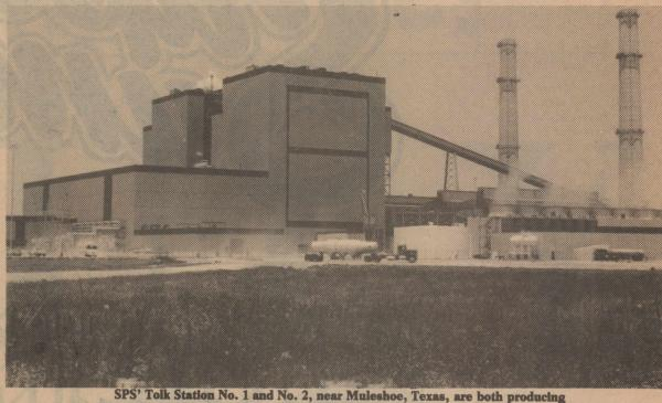
SPS' Tolk Station No. 1 and No. 2, near Muleshoe, Texas, are both producing electricity now. Wyoming coal is burned in steam boilers in the 20-story-tall boilerhouses, center. Then Steam flow drives each of the 561,000-kilowatt turbine- generators, which produce the electricity. The boiler flue gasses are cleaned in baghouses before exiting 400-foot stacks, right. [SPS photo]
