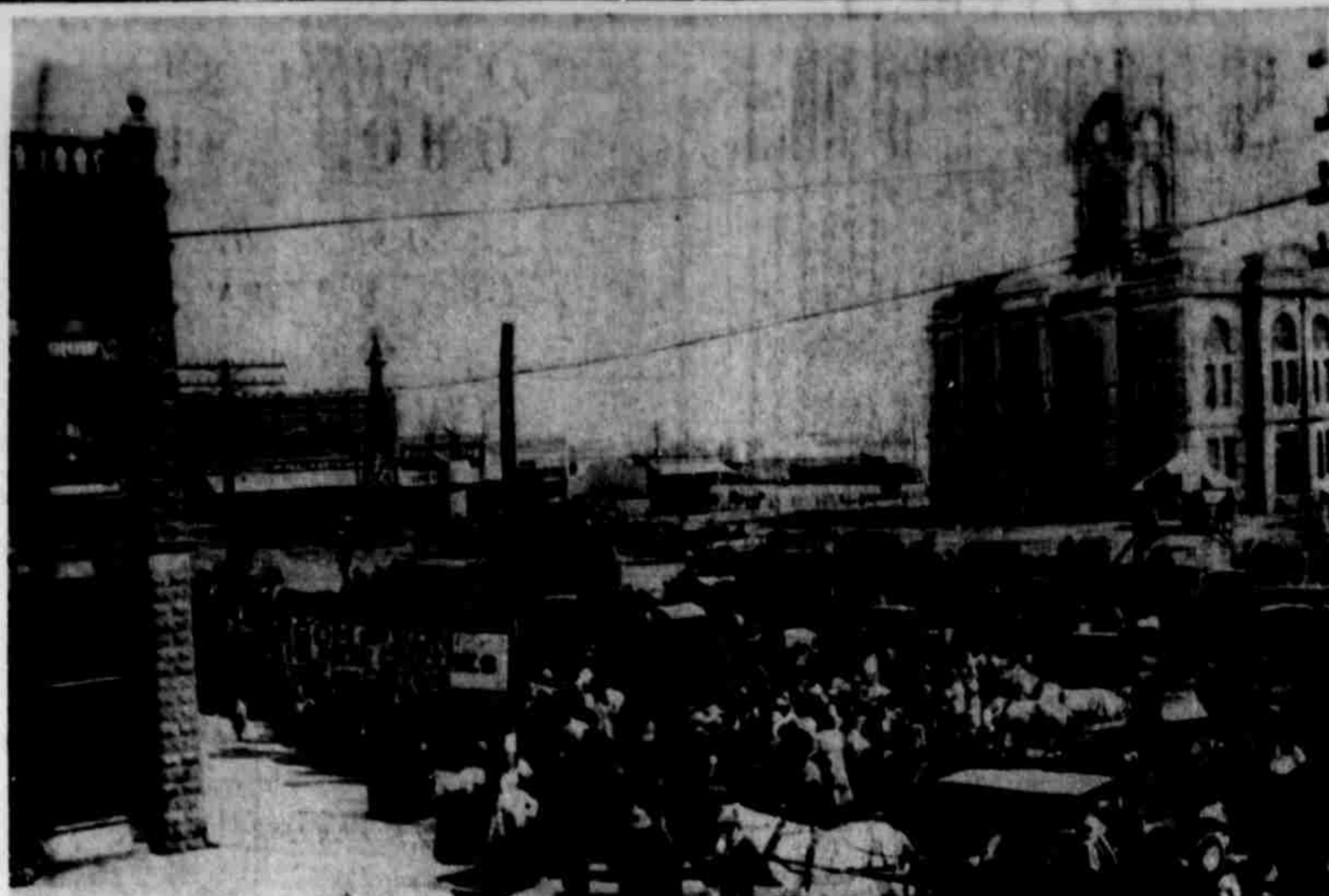
AN EARLY DAY STREET SCENE in Haskell, believed to be about 1906. Taken from the North-west corner of the Square.
