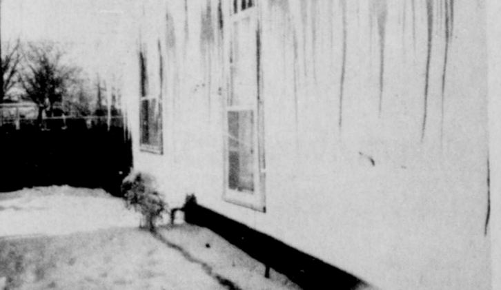
ICICLES formed the full length of the house above, with some of the ice hanging down from the roof more than three feet long.
