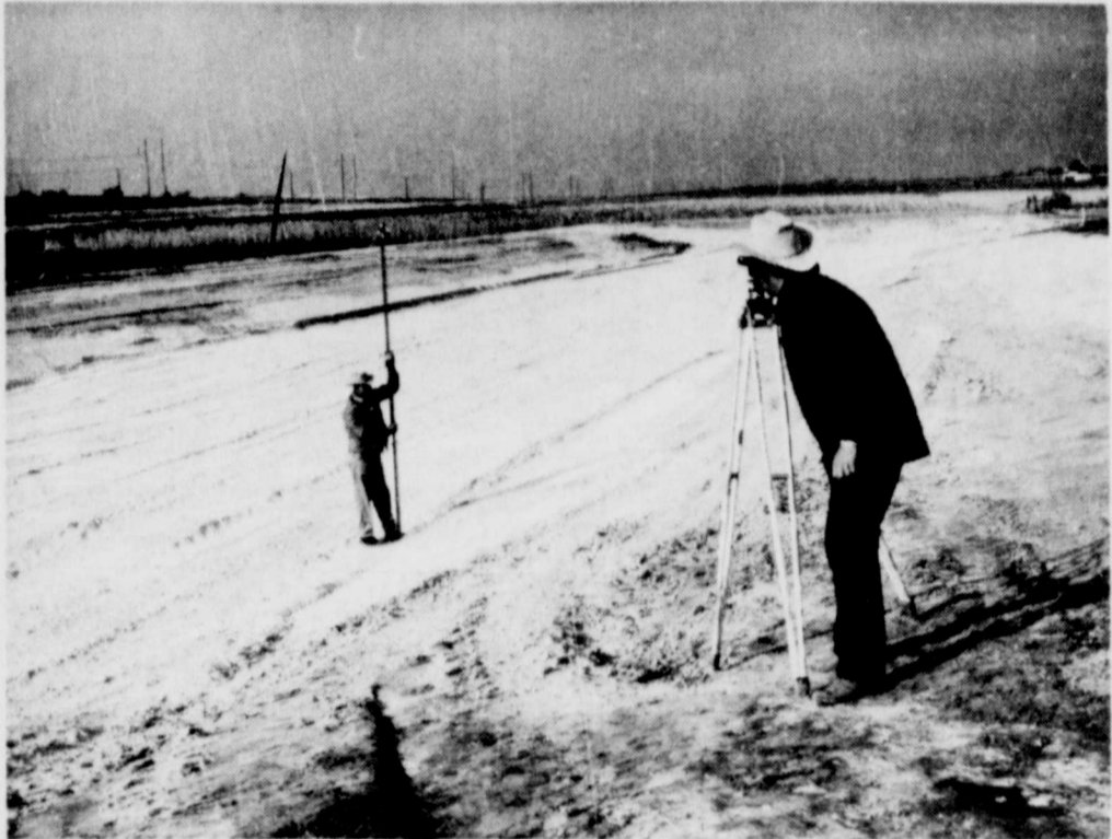
TECHNICAL HELP—Staff members of the Soil Conservation Service are shown furnishing technical assistance in the construction of a pollution control pit at Lubbock Christian College's 4,000-head cattle feedlot about four miles north of the city limits. The pit will store runoff from the biggest rain that can be expected in a 24-hour period (5.2 inches) in 25 years. Costs of constructing the pit and diversion terraces above it are estimated at $5,000. Feedlot wastes that collect in the pit will be pumped onto 100 acres of Midland Bermudagrass. (SCS Photo)
